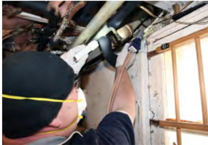
Advantage Weatherization worker seals air leaks in a basement to help stop drafts.
